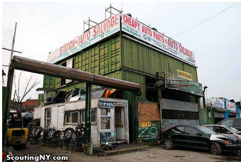
Exterior of Shop Made of Shipping Container
