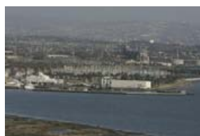
Aerial view of the South Bay Power Plant.
